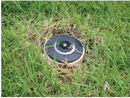
Fig 7: A typical pop-up sprinkler head when not in use (left pic) and when in operation (right pic).
