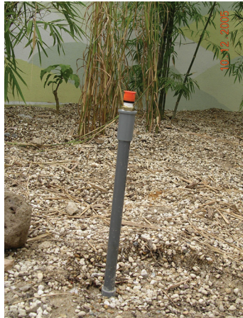
Fig 8: A permanently raised sprinkler head.
