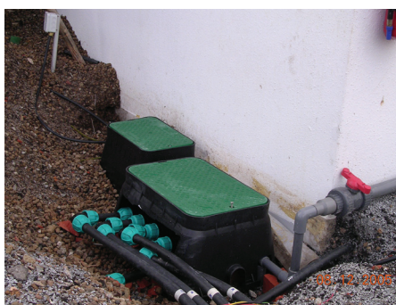
Fig 6: A typical valve chamber in a semi-buried box (left pic) and the valves inside the chamber (right pic).
