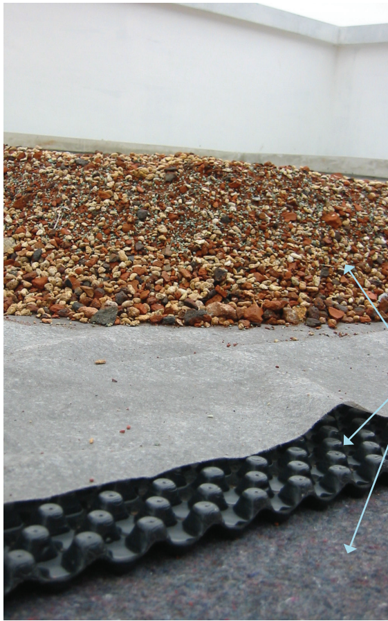
Fig 5: The locations where water is stored within a typical extensive-type green roof system.
