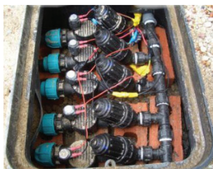
Fig 6: A typical valve chamber in a semi-buried box (left pic) and the valves inside the chamber (right pic).
